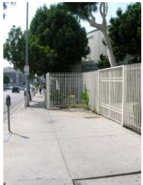
Overheight, wrought-iron fencing overdefines the division between public and private realms and creates a harsh, forbidding outdoor environment .
