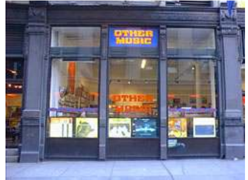
This window sign identifies the business while not obstructing views into the display windows.
