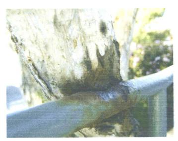
The photos above show the existing trees lining the entrance of the school. As you can see, these trees have been seriously damaged and they are damaging the existing railing system. We plan to remove the railing system and to replace these trees with the California Bay Laurel (Umbellularia Californica).
