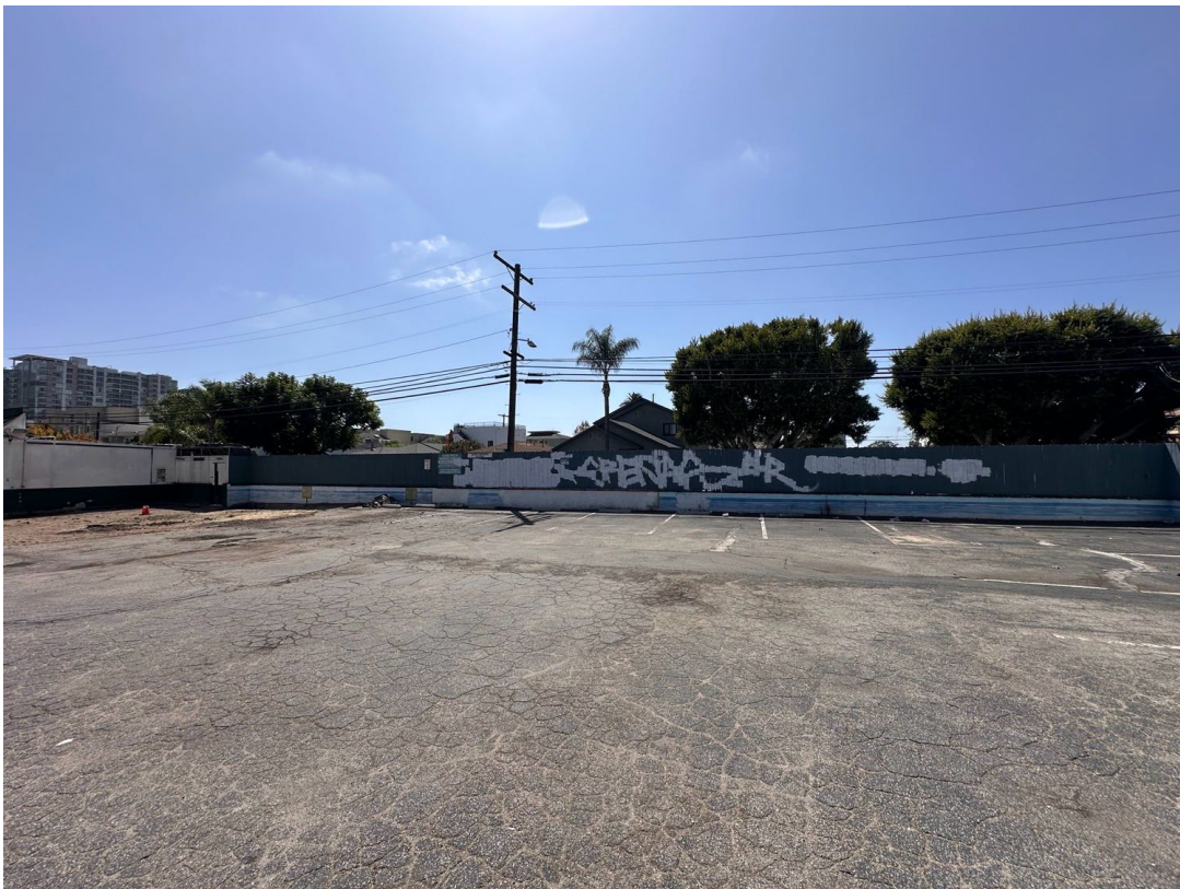
Photo D--Parking Lot looking west toward Carter Avenue. The existing wood fence on concrete retaining wall forming the west boundary, with homes immediately behind.
