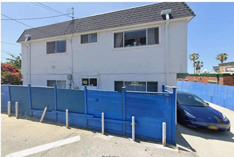
View of East elevation along Speedway Ave.
