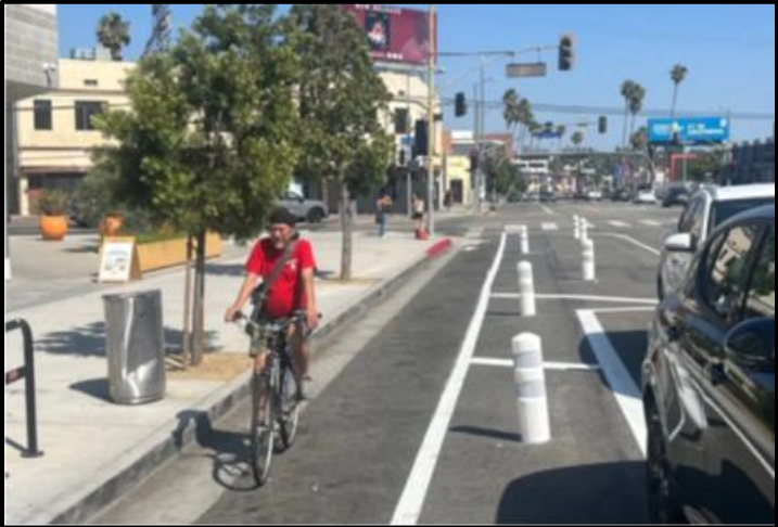
Figure 6: Protected Bike Lanes along Broadway Avenue, Santa Monica
