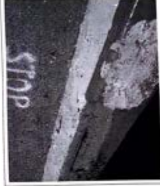
Dell Photo 2: Large concrete spalling section with subsurface exposure
