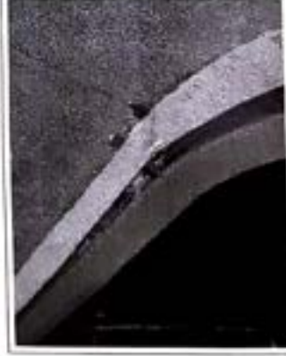
Dell Photo 1: Concrete parapet base — cracking, joint delamination along joint
