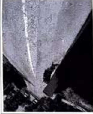
Dell Photo 2: Large concrete spalling section with subsurface exposure
