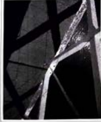
Photo 9: Mineral deposits, cracked deck boards, rebar corrosion
