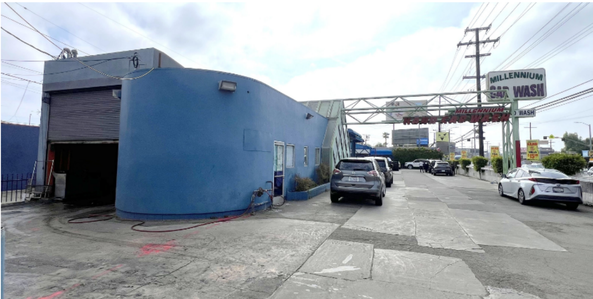
EXISTING BUILDING PERSPECTIVE - NW CORNER
