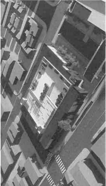
AERIAL VIEW - WEST BUILDING
