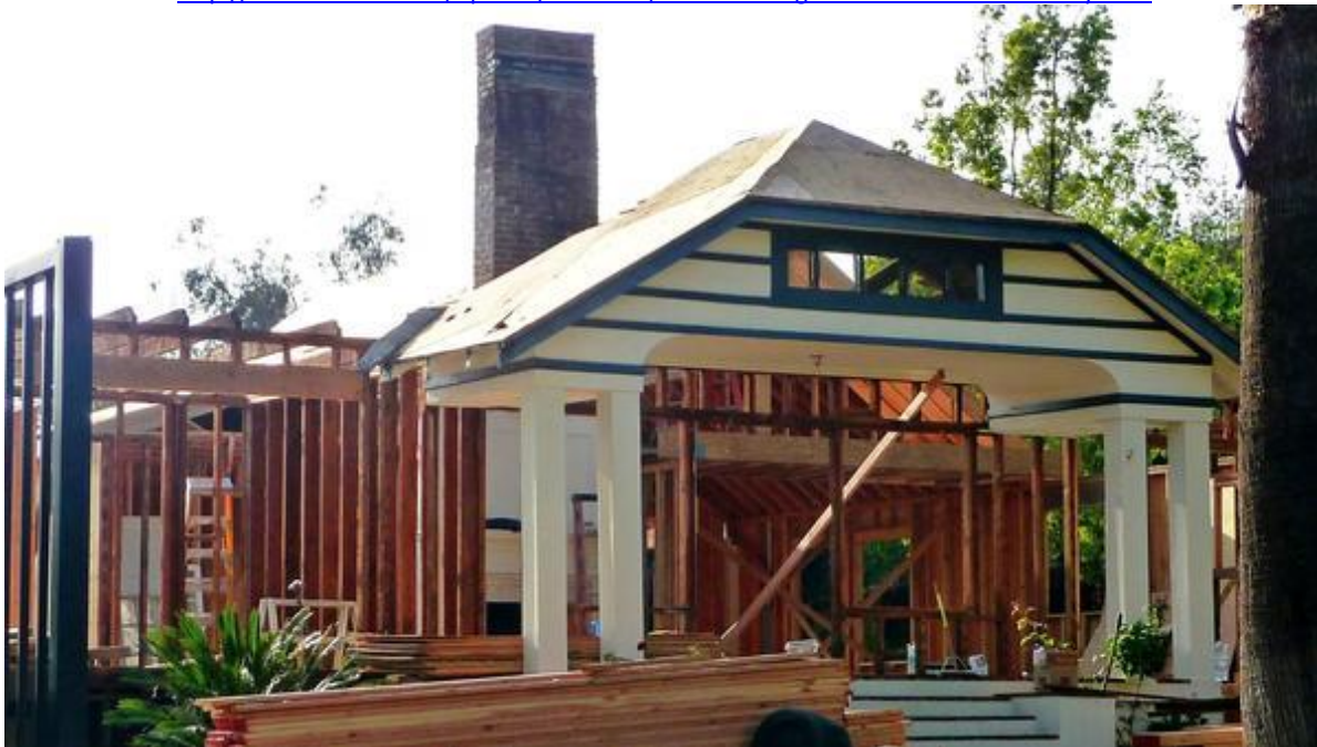
Only the porch and facade remain during a reconstruction of this 1930s Craftsman home, located in La Cañada Flintridge, on Feb. 7.
