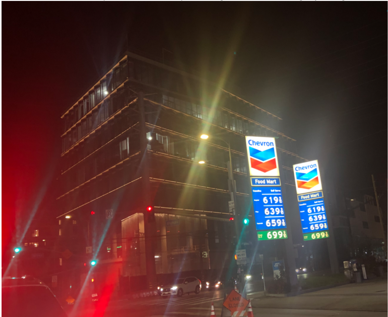
WestEdge project (Olympic Blvd., old Martin Cadillac site): Horizontal light bands that shine into houses to the south.
