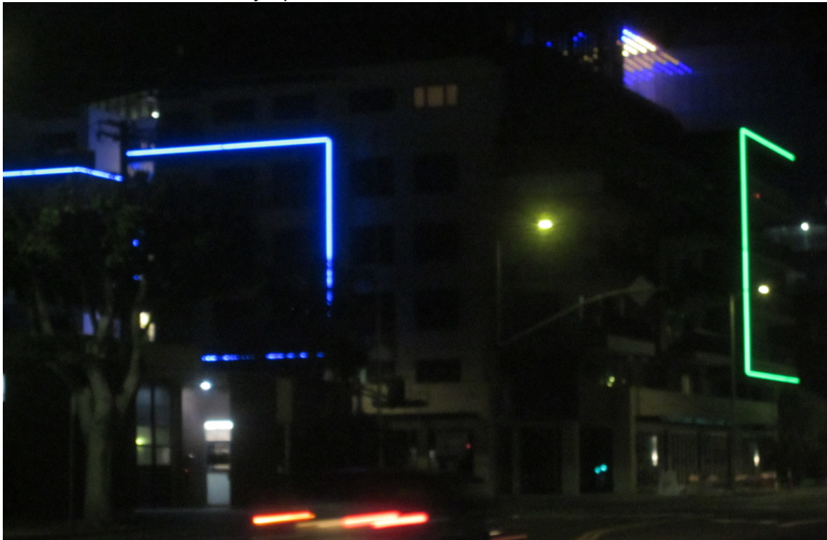
Olympic / Butler project: Neon on side of building that shines into houses to the west.
