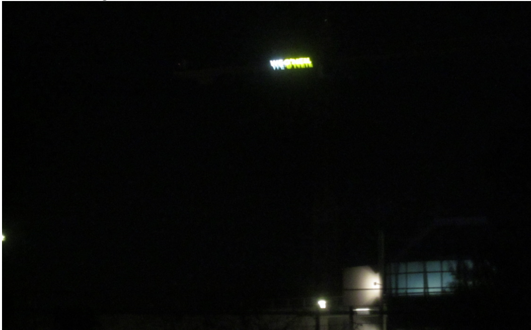
West Edge project (Olympic / Bundy): Construction crane facing south and shining into residential neighborhood (O'Neill Construction).
