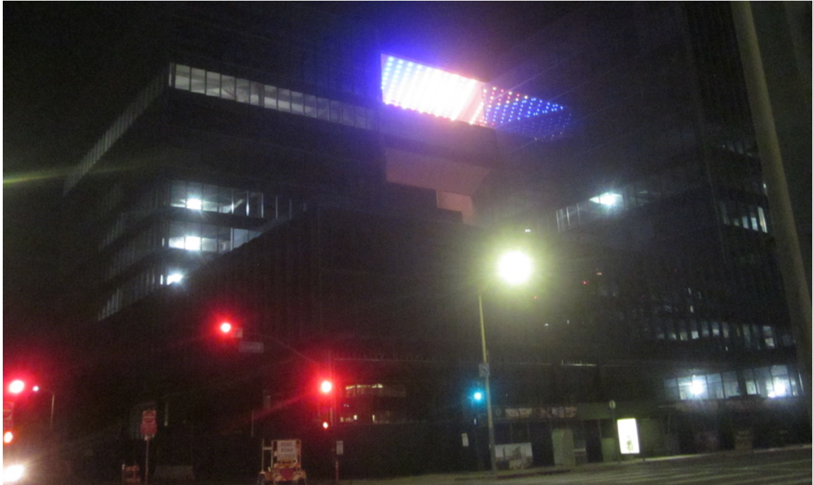
Lumen project (Olympic Blvd.): LED lights (colors, flashing) on bottom side of pavilion on roof that shine onto Olympic and houses to the north.
