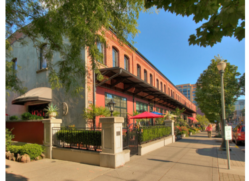
Awnings, umbrellas, and enclosures break down a long building frontage and help create a human-scaled frontage at the sidewalk in Portland, Oregon.
