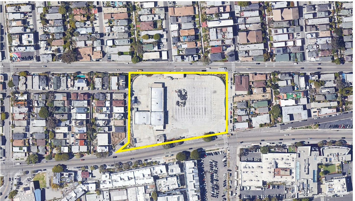
Aerial Photo of Existing Conditions, Google Earth, 2018
