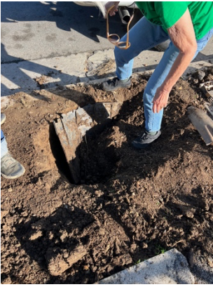
Digging out old buried tree root guards and tree roots
