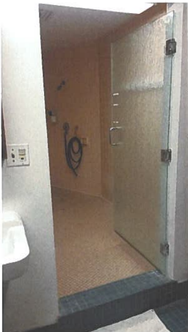
Non-conforming threshold
