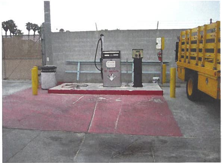
Existing diesel fueling station
