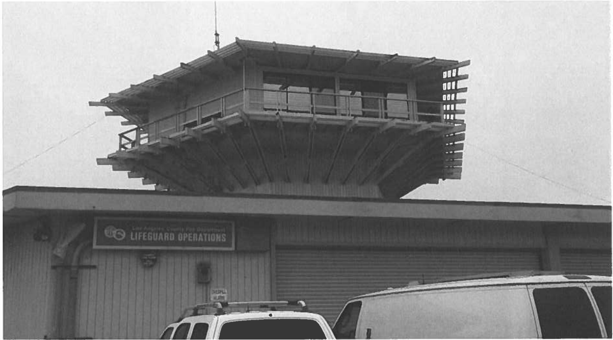
View from service yard looking west at Northeast building elevation
