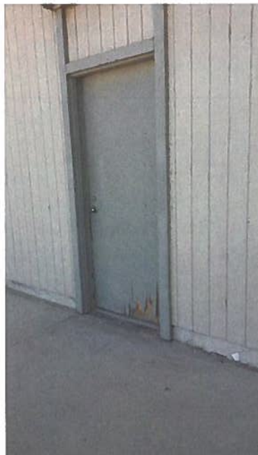
Condition at exterior door
