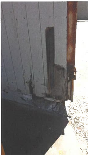
Condition at building corner
