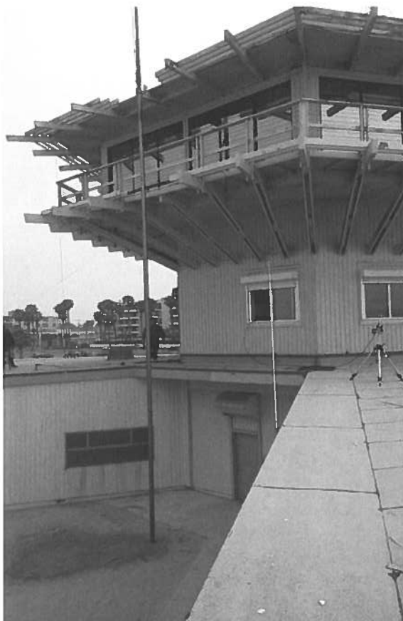
View from lower view looking at southwest elevation
