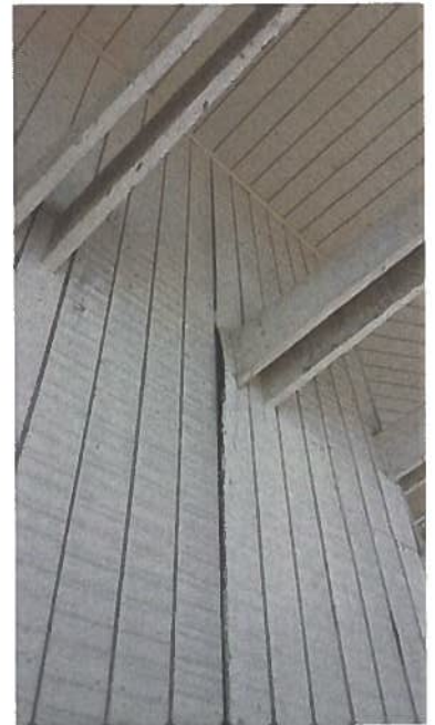
Condition at 2 nd level wood siding
