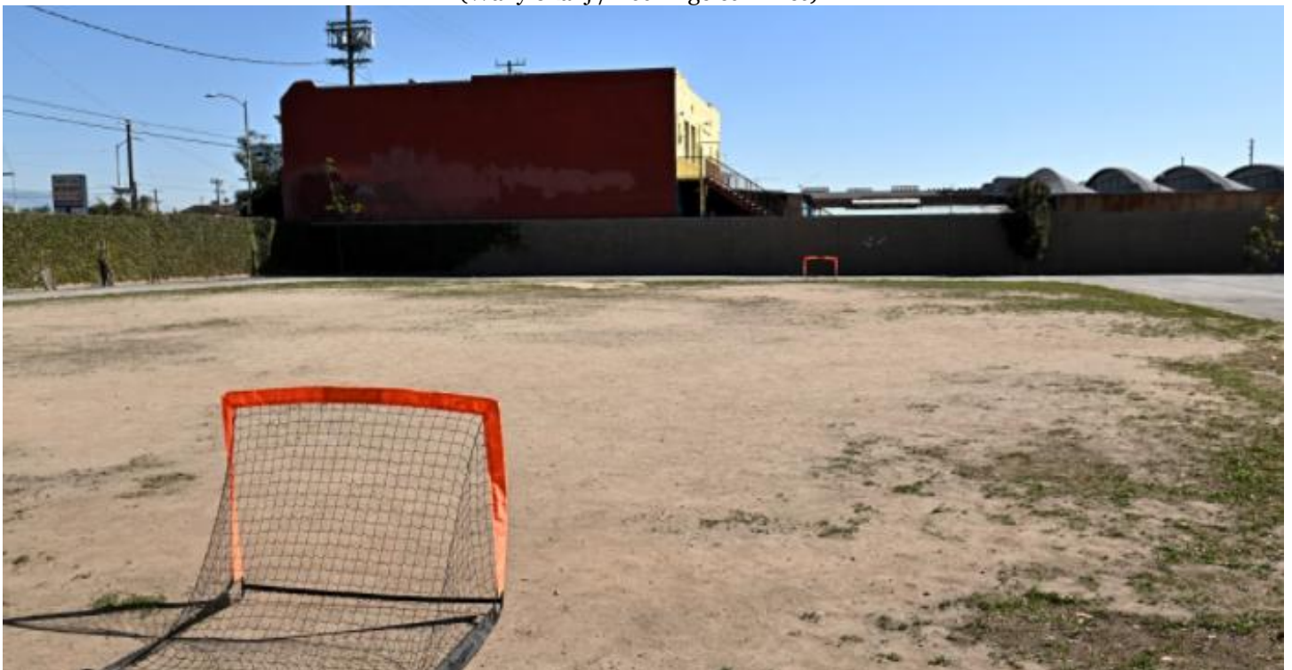
A play area at Castellanos Elementary in Los Angeles that lacks a working sprinkler system. (Wally Skalij / Los Angeles Times)
