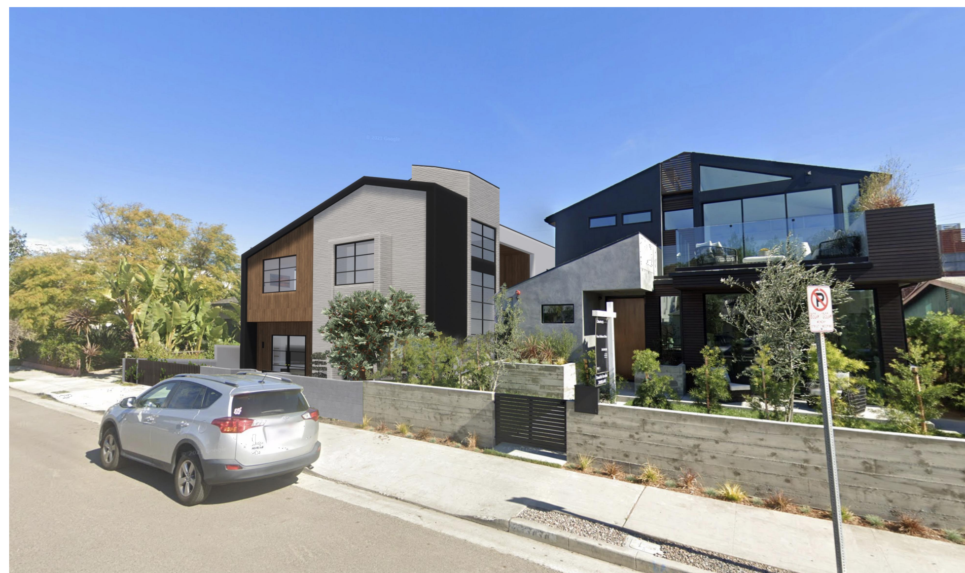
B - SIDE APPROACH STREET VIEW FROM CLOY AVE
